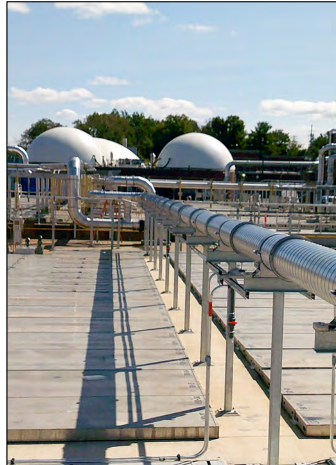
Odor Control Duct for Primary Settling Tanks ##1-6 taken (09/18/20)
