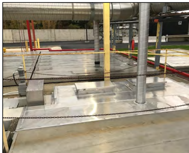
Primary Settling Tank #5-east Cover Installed taken (10/29/21)
